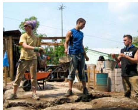
7. Hand carry the wet concrete to the footings.
