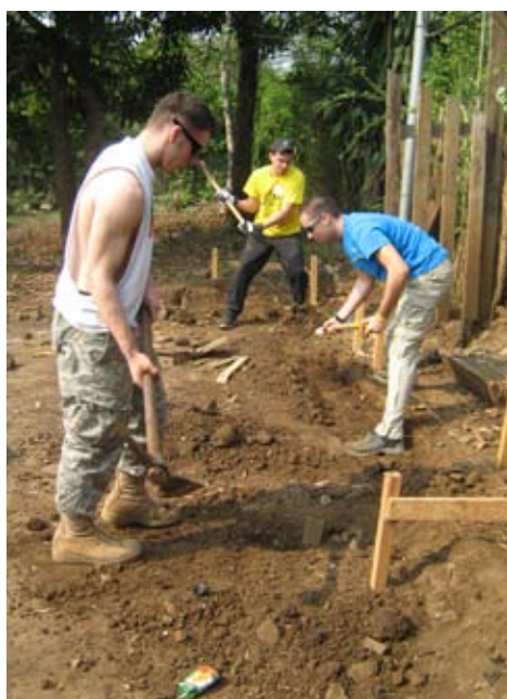
2. Dig the footings.
