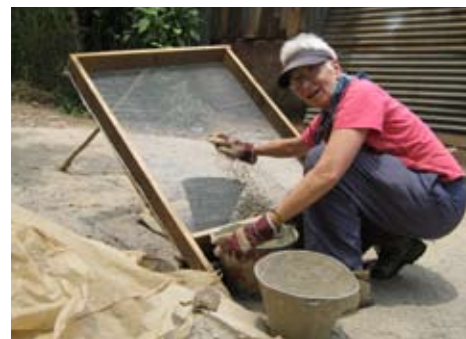
5. Sift by hand the sand to get a consistent texture.
